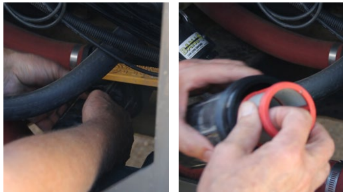
Unscrew the supply water filter.
