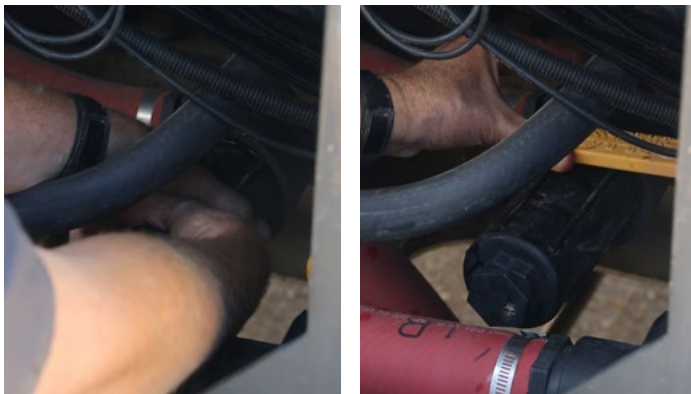
Close the supply water isolation valve.
